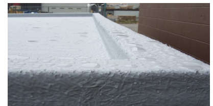
Fiberglass pan (above) holds spilled liquid, it is mounted to modular building and then sealed with fiberglass for seamless flow from floor to ceiling.
