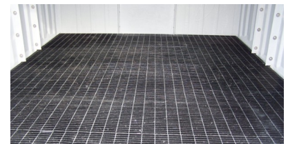
Fiberglass pan (above) holds spilled liquid, it is mounted to modular building and then sealed with fiberglass for seamless flow from floor to ceiling.
