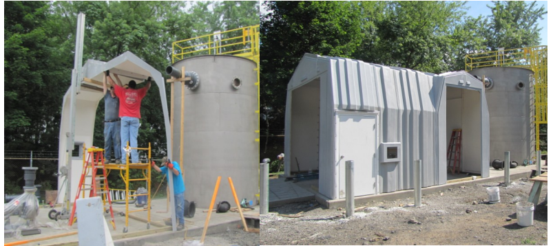
A Local contractor assembled the RM Products modular fibreglass building onsite around existing equipment at the Borough of Ashland Waste Water Treatment Plant in Pennsylvania .
